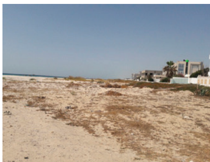
Figure 3. The pressure of the building on the beach of Menzil Temime. Photo: Hagui A., Najem D., 2020.
